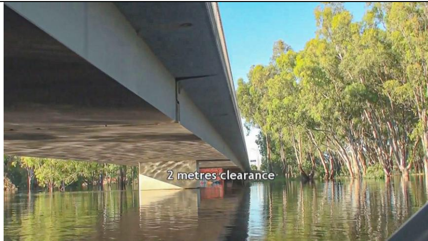
Plate B5.3 – Hay Bridge clearance (Source: Mr. R Shiller)
