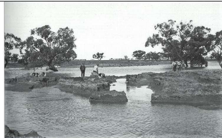
Plate B1.4 – Making a start on the task of repairing the Bungah Creek washaways after the flood damage in July 1931. (Source: Hay Historical Society)
