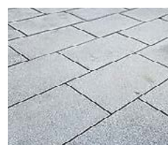
300 x 600mm appropriately textured feature granite paving surrounding Witcombe Fountain and other monuments and public art pieces.
